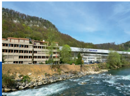
HAEUSLER headquarters in Duggingen, Switzerland
