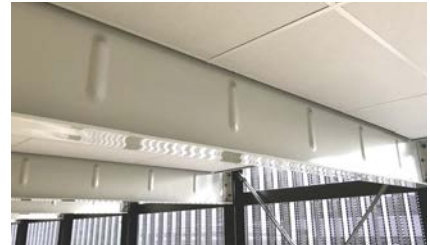
112 Add beam stiffener with the Stierli press
